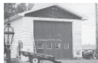
Shop's insulated door consists of two 16 by 8-ft. sections hinged across the middle.
